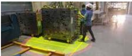
Mounting on crane
